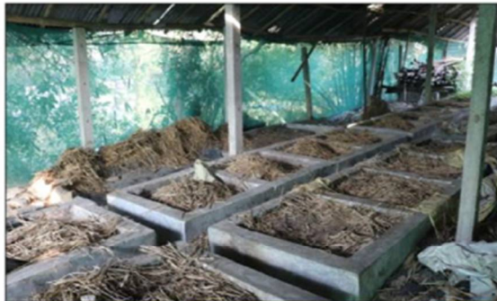
Construction of Vermicompost Pit
